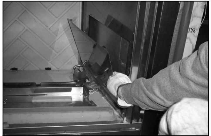
Figure 6.4 Remove Valve Access Panel
